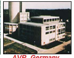
AVR, Germany 15 MWe, 1967-88
