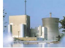
THTR, Germany 300 MWe, 1986-89
